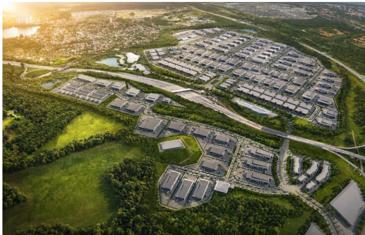
Elmina Business Park 2 (Industrial lots) 19 units | RM260.4m
